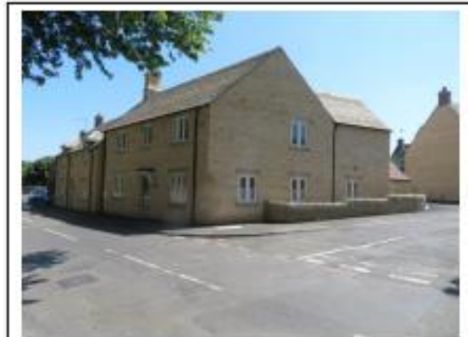
School Road, Barnack
